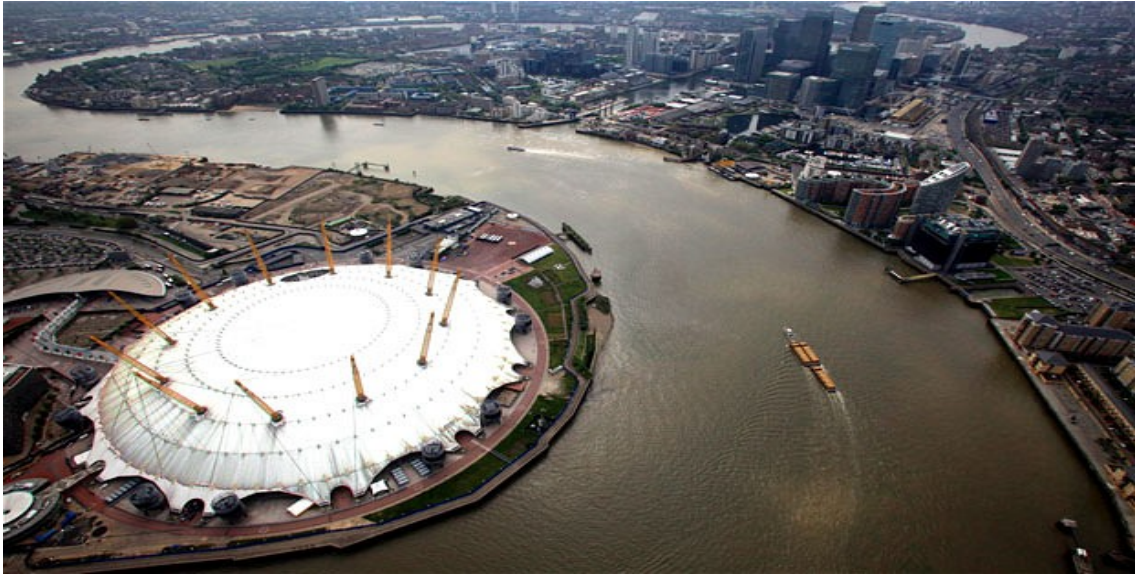
Fig. 6.2 The Millennium Dome 32
