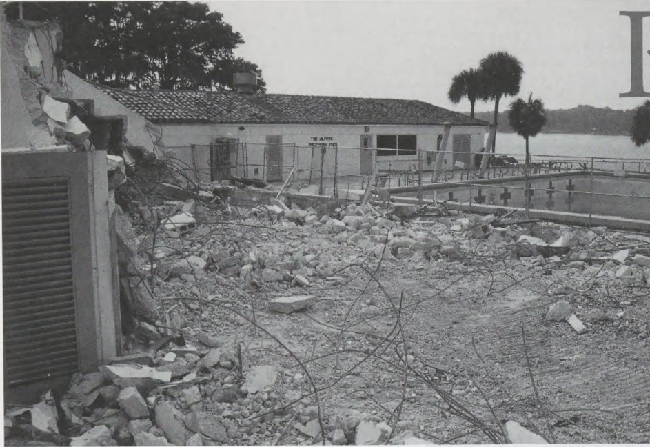
View of Alfond Pool House following the demolition of the bleachers
