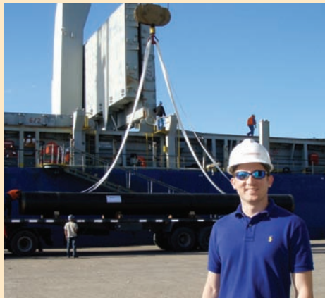
McCarthy on a recent trip to Argentina. In the background, pipes are being unloaded for the Natural Gas Pipeline.
